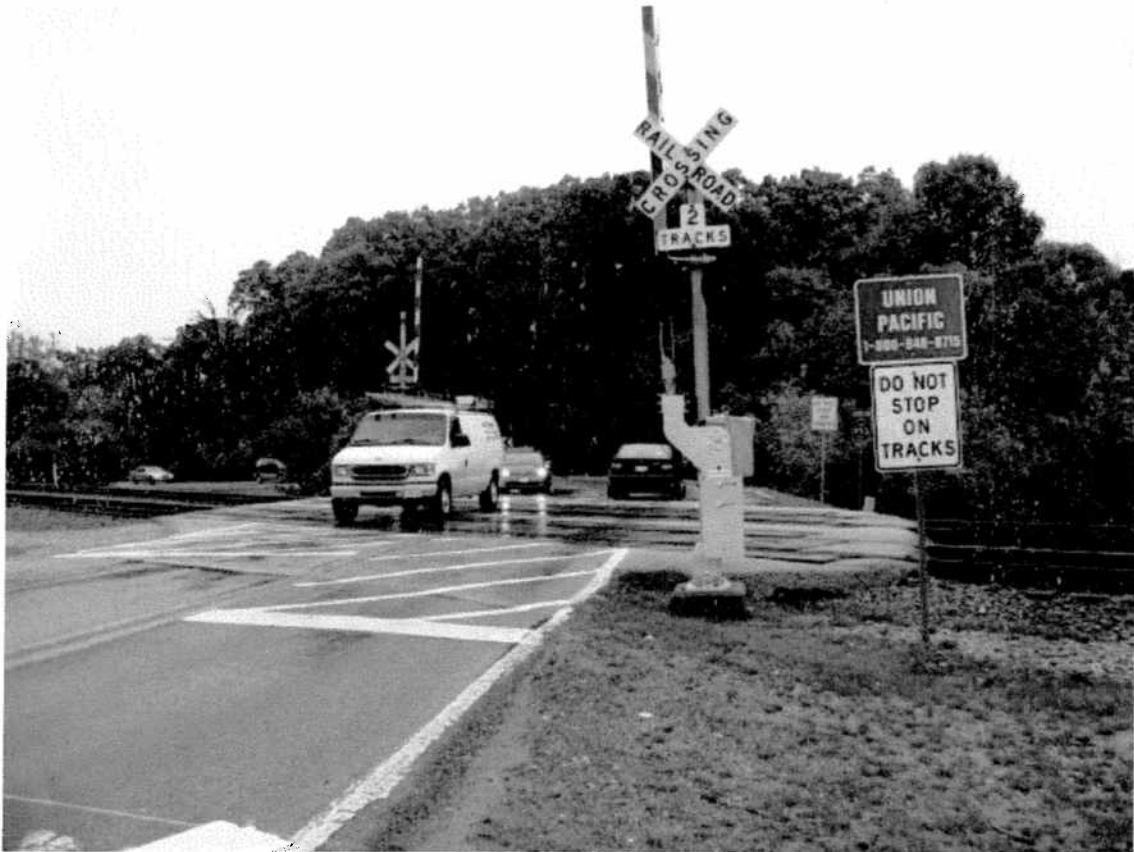
Union Pacific Crossing, Hart Road – Looking South
