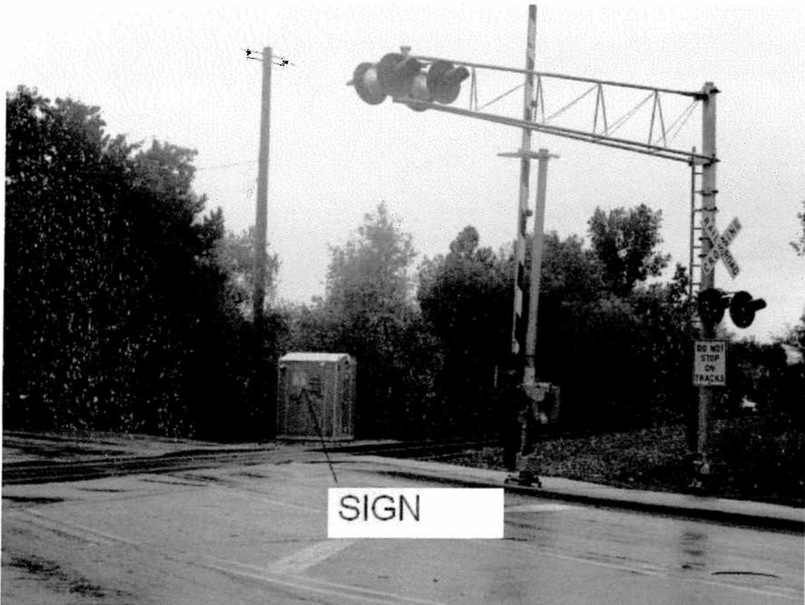
EJ&E/Canadian National Crossing, Hough Street – Looking South
